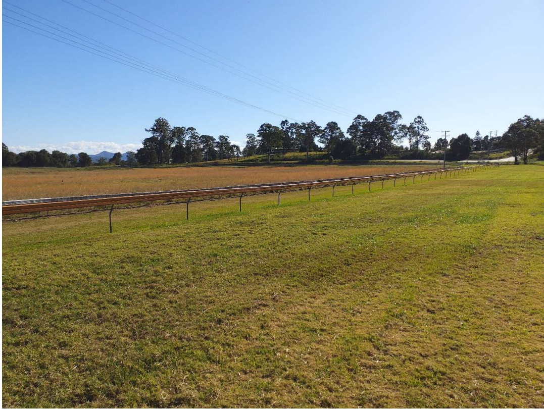
Fence going to be replaced
