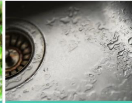
SMART WATER ADVICE A drip a second wastes 12,000 litres per year.
